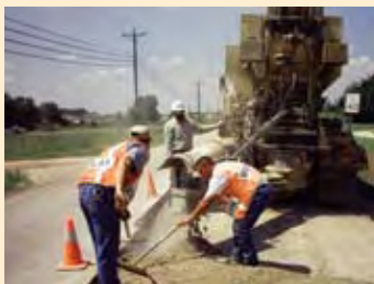
Our concrete is mixed on site, so it's always fresh.
