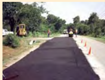
Road is open 4 hours after pouring.
